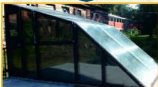
Head based storage Solar Kiln
